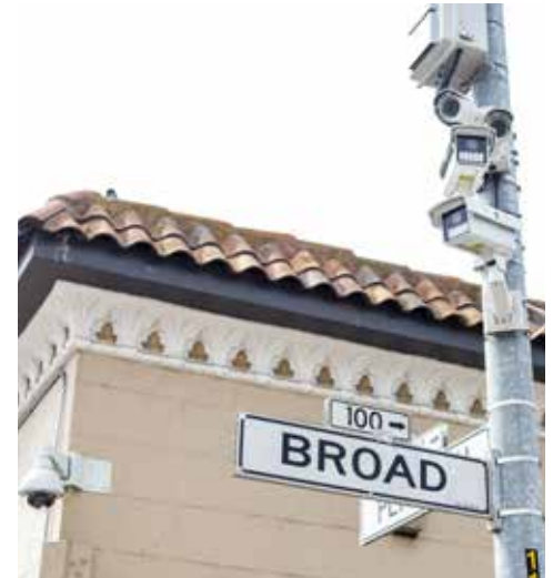
New cameras installed at the Plymouth/Broad intersection.
