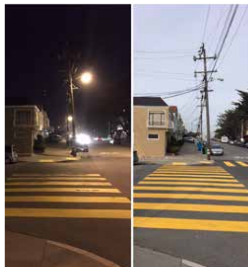
Before and after painted crosswalks along Quintara.
