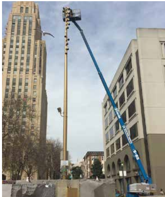
The lights at the UN Plaza fountain are replaced.
